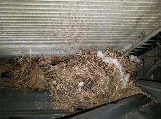
A cause of premature condenser failure is excess debris in and/or surrounding the condenser.
