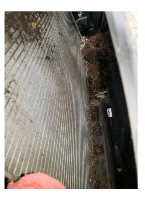
Extend the life of your condenser by cleaning out excess debris surrounding the system.
